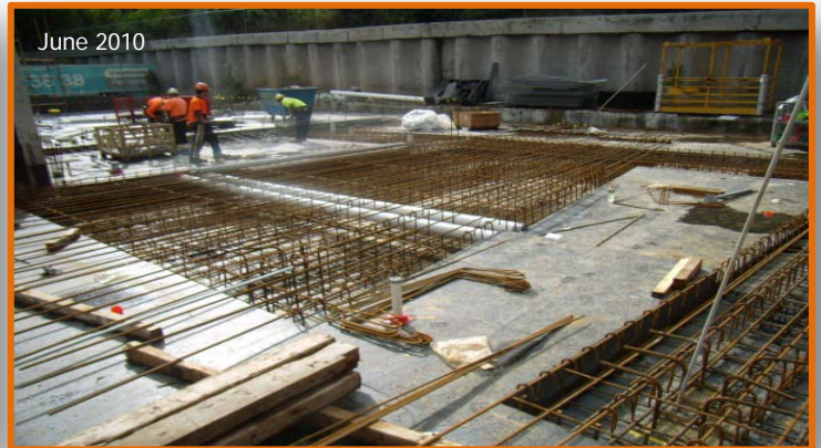
Building C - Transfer Beams to Level 1
