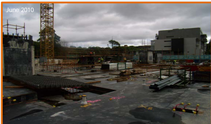
Building C Level 1- Formwork in progress
