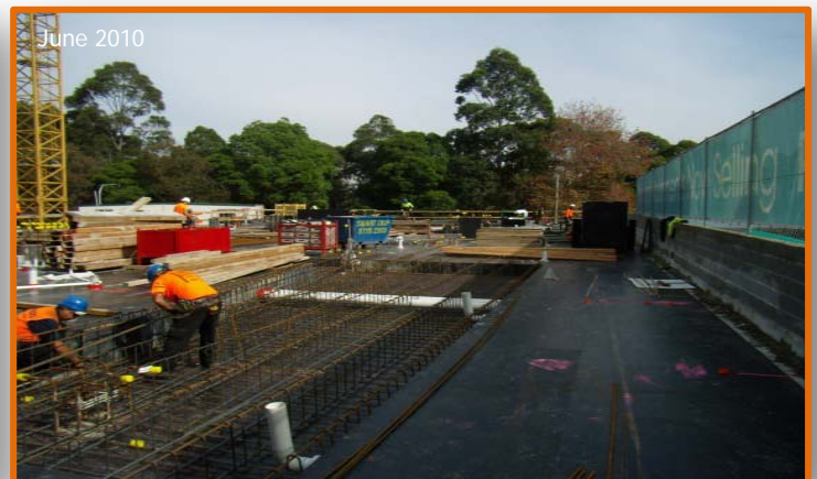
Level 1 Podium Slab Between Building B & C
