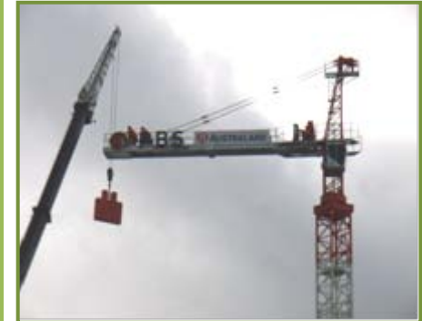
Step 4 Counterweight & Struts
