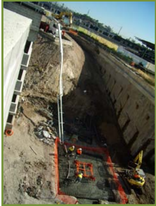
Step 1 Crane Base Concrete Basement
