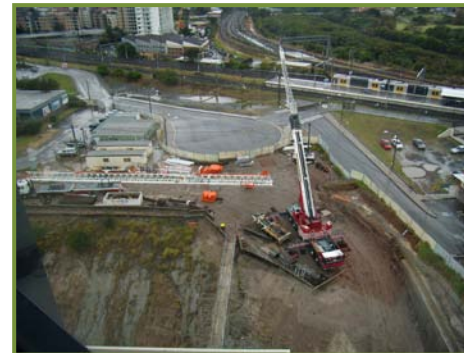
Step 3 Mobile concrete pump
