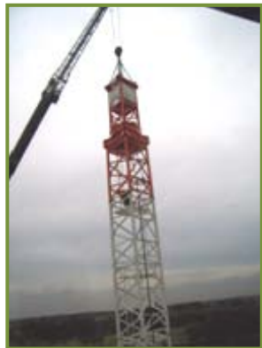
Step 5 Slew Ring & Cat Head Installed
