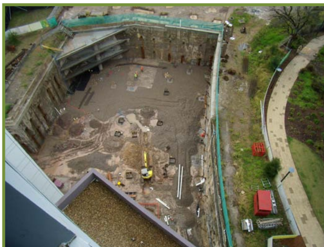
Site preparation prior to Crane Tower erection
