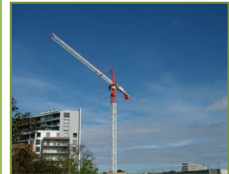
Step 8 Crane Commissioned
