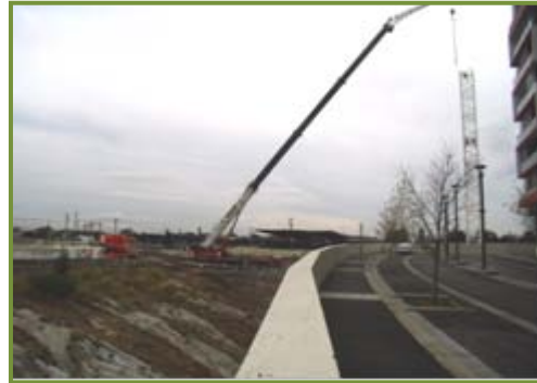
Step 2 Tower Erection
