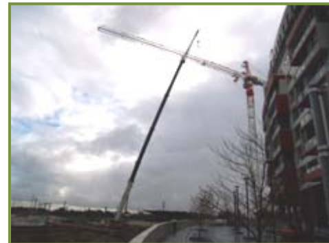
Step 7 Main Boom Installation
