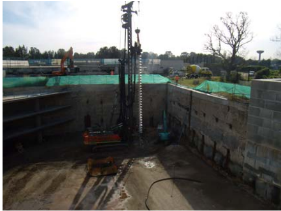
Drilling rig with 20m auger
