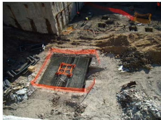
Tower Crane base foundation
