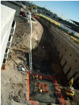
Concreting of Tower Crane base foundation
