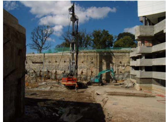
Drilling for pile foundations
