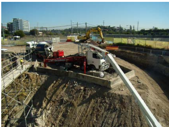
Mobile concrete pump
