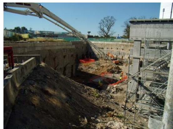
Mobile concrete pump with extended boom to reach bottom of basement
