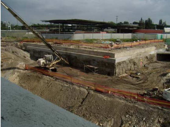
Installation of soil anchors by drilling rig
