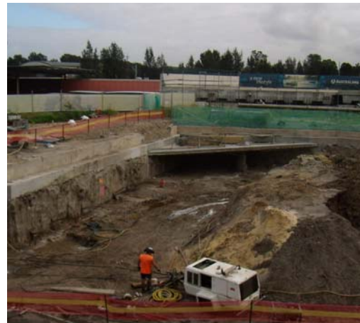
Bracing slab acting as wedge
