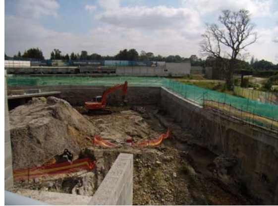
Excavation of basement by hydraulic excavator
