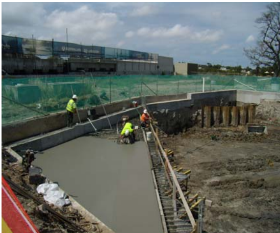
Pouring of bracing slab
