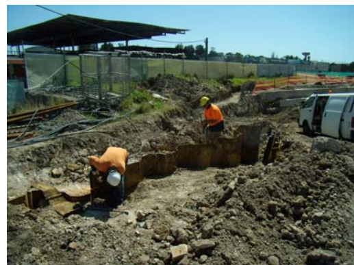
Removal of buried sheet pile
