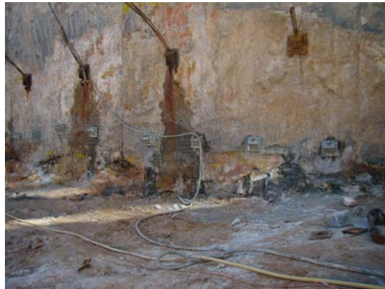
Rock bolts (silver) and soil anchors (brown) installed in diaphragm wall
