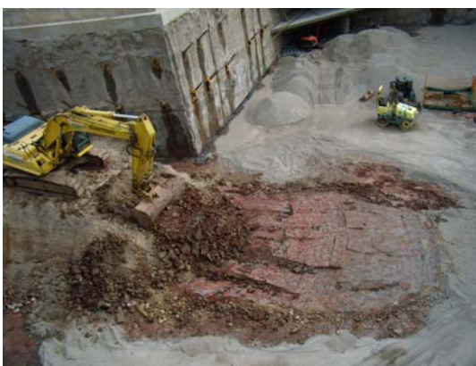
Trimming of temporary ramp
