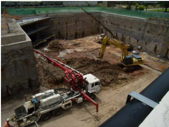
Concrete pumps, excavators, drill rigs ....it's all happening!
