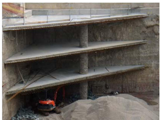
Excavation under final bracing slab
