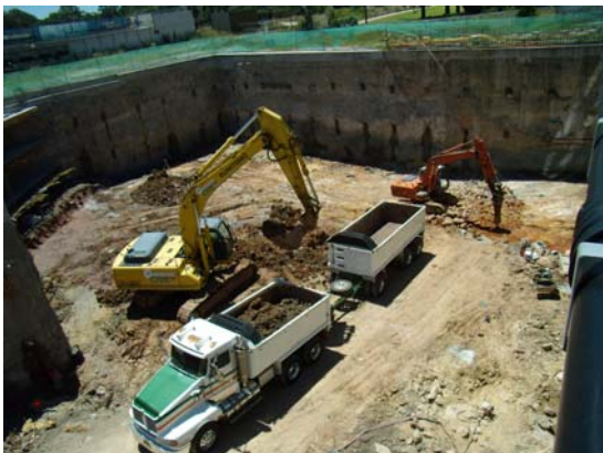
Trimming of final bulk excavation level
