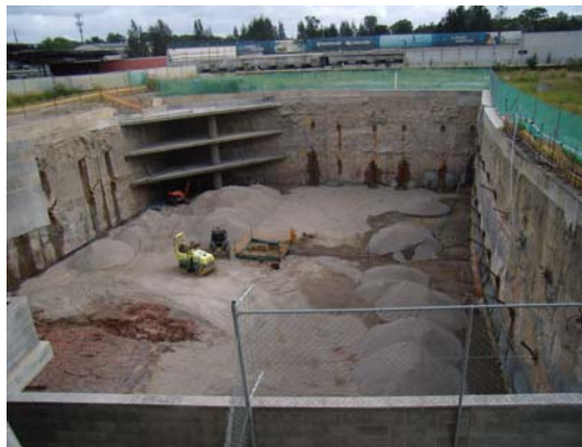
Placement of crushed rock base
