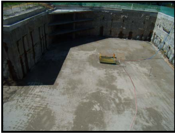
Completed Bulk Excavation
